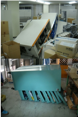
Figure 2: Many electronic racks and tool boxes which were not fixed fell down.
