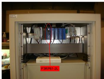
Figure 6: The F3RP61-2L (the second left module) serving as an EPICS IOC to control a pulse magnet power supply.
