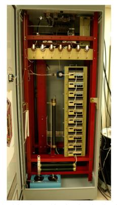
Figure 4: High voltage cabinet interior, showing the solid state switch (R), consisting of ten 3.3 kV switch modules connected in series.
