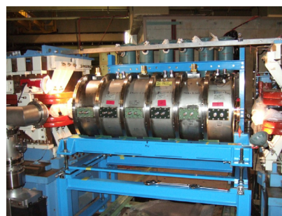
Figure 1: Induction cells installed in KEK-DA ring.
