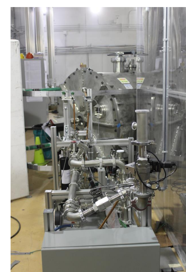
Vacuum & Gas Control: Modbus PLCs
