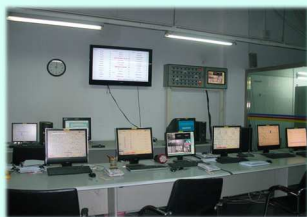
Cryogenic Control Room
