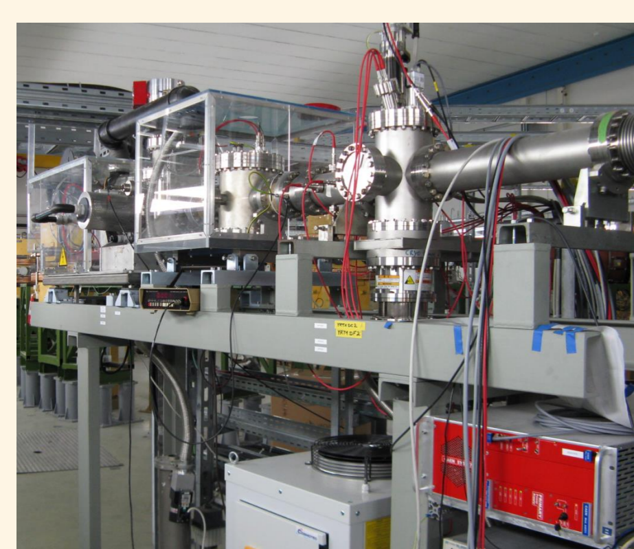
MINIS ion source platform (50kV) and Low Energy Beam Transfer (LEBT) with installed CAEN HV (red) for Einzel lense and electrostatic elements.
