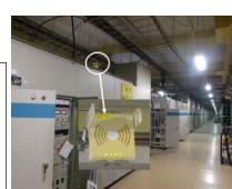
FIG. 6: Photograph of Access point for klystron gallery. Aruba-AP65.
